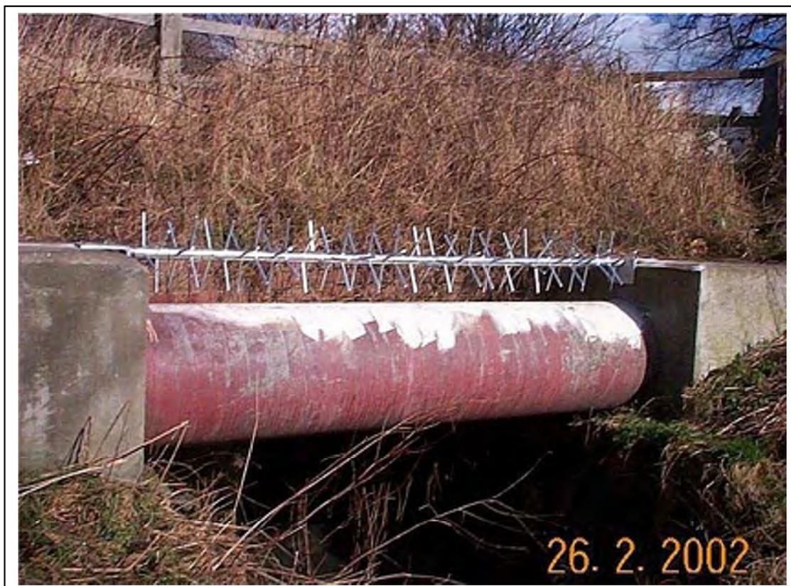
Care must be taken to ensure that the pipe crossing is capable of taking the increased structural loading imposed by any protective device.
